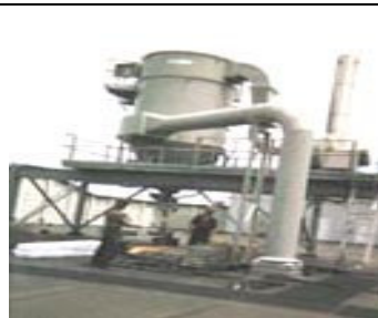
Roof Top Units
